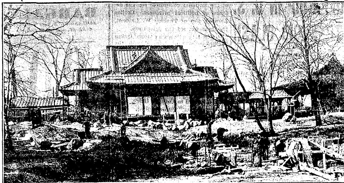
The picturesque Japanese buildings of the World's Fair of 1893, which have stood on Wooded island in Jackson park for forty-one years, are being restored by the south park board with the aid of public works administration funds.
